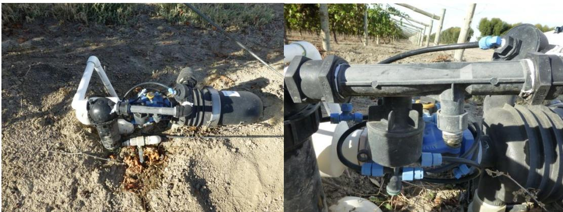
**Figure 1 Mazzei Venturi air injection system<sup>1</sup>**
